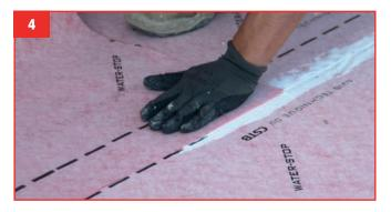
**4.** Fit the following strips of sheet leaving the joints unattached. The gluing and sealing of the joints will be carried out after the sheet has been placed on the entire surface.
