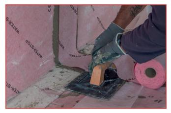
The waterproofing must extend along the vertical wall up to a height of at least 20 cm above the roof protection. The extension can be carried out by lifting the piece from the floor or, preferably, by means of overlapping bands on the floor.
