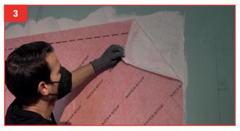
**3.** Lift a corner to check that the veil of fibres is completely covered with adhesive. If necessary, increase the amount of adhesive or correct the pressure.
