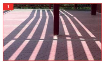
**1.** Check that the base surface has no uneven patches or debris that could pierce the sheet.
