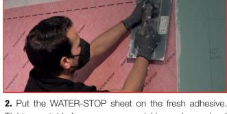
**2.** Put the WATER-STOP sheet on the fresh adhesive. Tighten, get rid of any creases or wrinkles and press hard from the centre to the edges with the smooth part of the trowel to expel air and excess material from underneath and achieve good adhesion.
