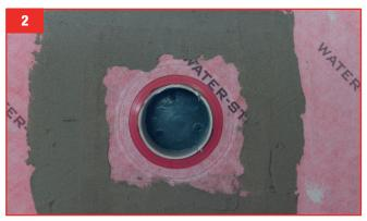
2. Prepare and treat particular points and items that will be connected to the sheet such as feeds to drains, expansion joints, pipes etc
