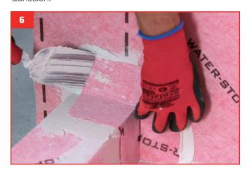
**6.** Check and ensure critical points are reinforced: corners, where the floor and walls meet, expansion joints, etc. Use WATER-STOP fittings for the reinforcement treatment of corners, joints, vertical strips and pipes and recommended sealing materials.
