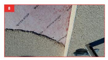
**8.** Once it has passed the water test, and any loss of watertightness has been dealt with, place the tiling or surface by gluing it directly on top of WATER-STOP.
