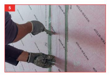
**5.** Glue and seal the joints between sheets. To ensure the sealing of the joints you can use W-S SEALMORTAR (or similar) elastic waterproof cement, W-S MASTIC adhesive and sealing putty (or similar) or W-S BUTIL butyl sealing tape.
