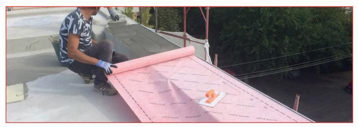
Then apply the cement glue, spreading it in sections and returning the sheet to its position to glue it by pressing towards the edge with the help of the smooth face of the trowel.
