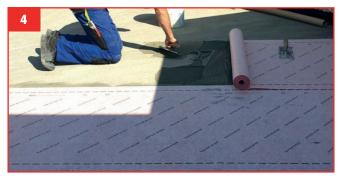
**4.** Glue the WATER-STOP sheet to the base leaving the overlaps and joints unclosed: spread the cement with the toothed trowel in parallel lines and apply the sheet on the fresh adhesive, pressing hard to achieve maximum adhesion.
