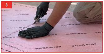
**3.** Prepare the sheets to the required measurements. Allow between 5 and 10 cm for the overlaps where sheets join and that the base sheet must rise up to 20 cm on the walls.
