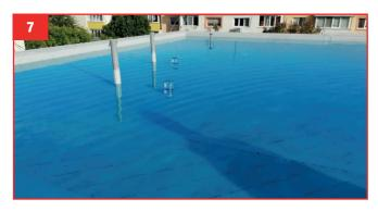
**7.** Whenever necessary, wait 8 to 24 hrs for the sealing material to cure and perform a water test to check that there are no flaws.
