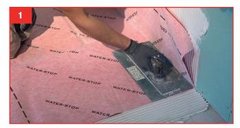
**1.** Apply to the surface to be covered by pressing with the smooth, plain part of the trowel to obtain maximum adhesion to the base layer. Spread in a layer of regular thickness making passes in one direction only with the toothed part.
