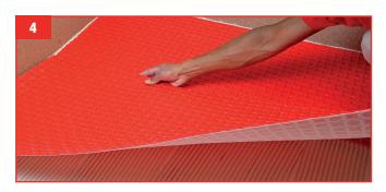
**4.** Then install the following pieces of G-Flex in the same manner. To ensure a flat surface, do not overlap the edges or ends of one m Z embrane over another. Spread G-Flex edge to edge with adjacent pieces without leaving gaps of more than 3 mm between membranes.
