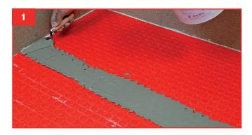
1. Apply EASEAL polymeric waterproofing cement centred in a 15 to 20 cm (6" to 8") wide strip.
