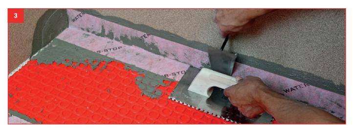
**3.** Place the W-S BAND on the bonding layer. First on the walls and then overlapping at least 6 cm (2-1/2") over G-Flex. Press with the smooth side of a trowel or spatula to remove air and excess material.
