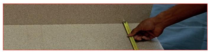
1. Cut G-Flex to the required size and shape, leaving a gap of 6 mm (1/4 inch) between the membrane and perimeter walls, columns, architectural elements, structural joints, drains, etc.
