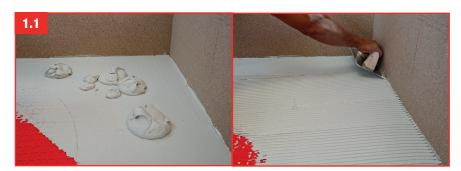
Apply an adhesive mortar suitable for the type of flooring. Use a tile adhesive with a minimum rating of C2 per EN 12004 or ISO 13007 or ANSI A118.4, ANSI A118.11 or ANSI A118.15.
